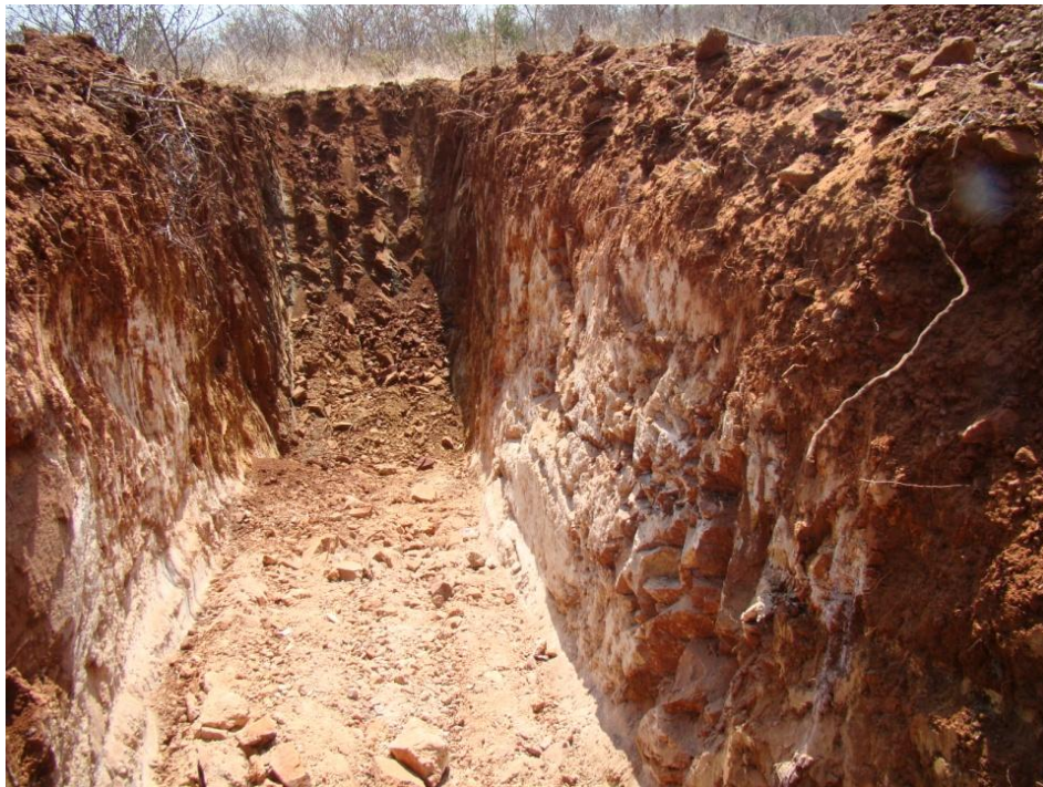
Figure 6 TR: A trench under excavation around the ATM workings
